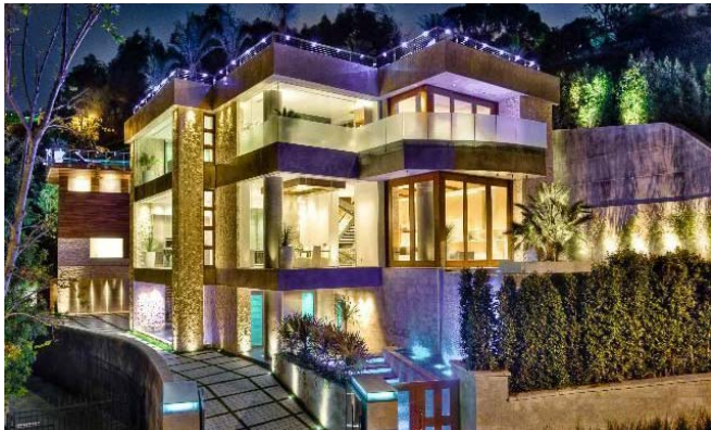
$15mm Beverly Hills house, Crestron controller, 120 switches, 40 keypads
